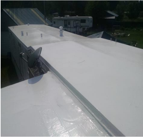
2015 Veteran Roof Coating Non Profit Project
